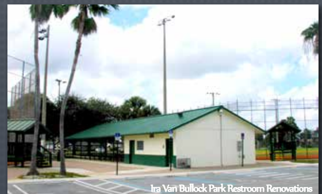
Ira Van Bullock Park Restroom Renovations
